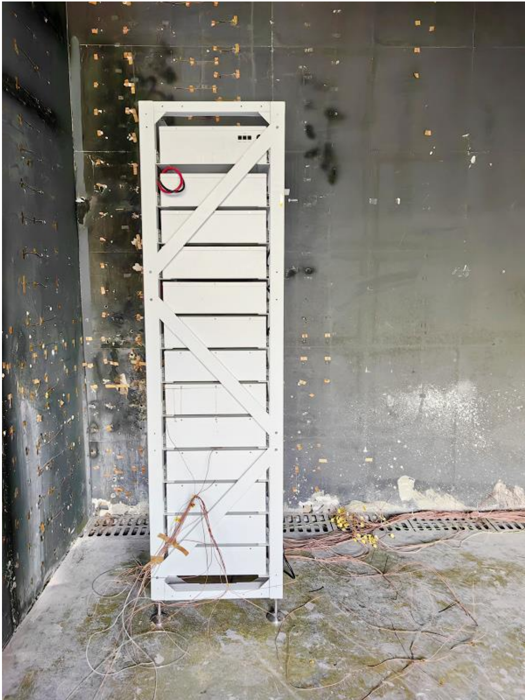
Figure 17. Photo 01 of initiating BESS unit after test.
